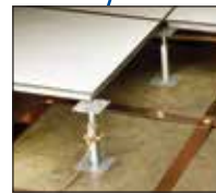
Signal Reference Grid (SRG)
